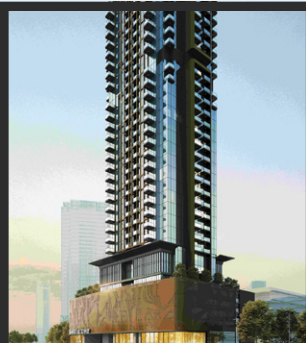
Seslia Tower JVT, Dubai
