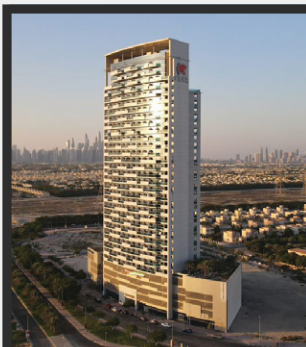
Al Jawahara Tower JVT, Dubai
